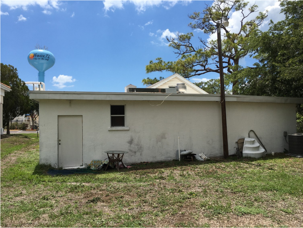
Rear view of church showing 1961 addition.
