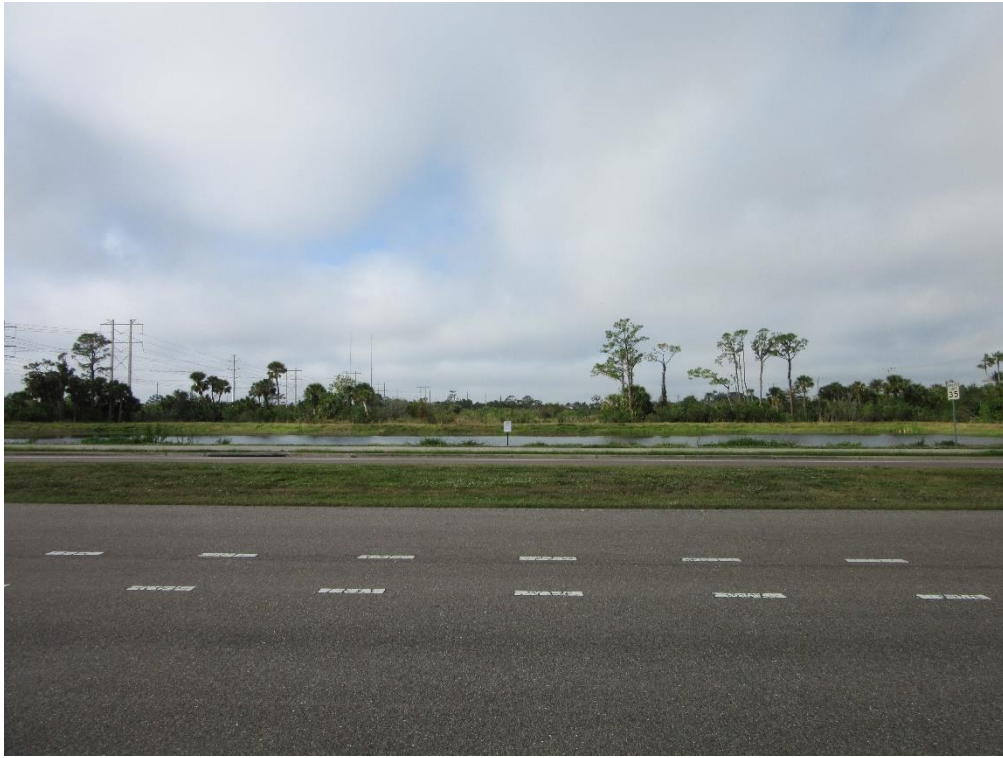
View to the West across Jacaranda Boulevard
