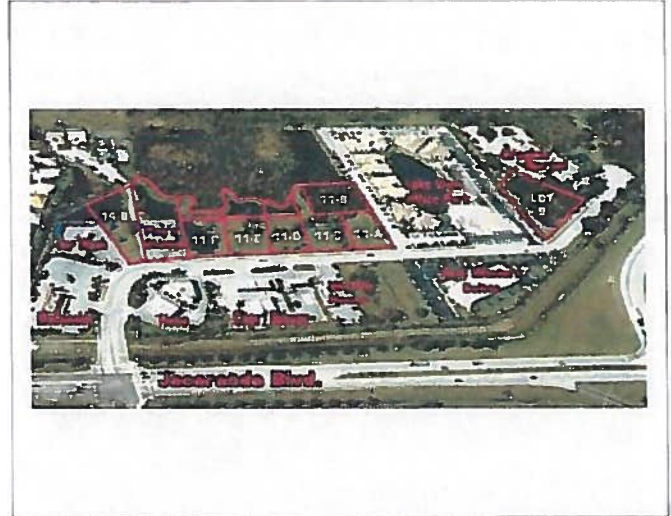
The Waterford Companies worked with Sarasota County to construct a deceleration lane and a new traffic signal located 1-75 and Jacaranda Blvd. Cost sharing for The Waterford Companies exceeded $300,000.
