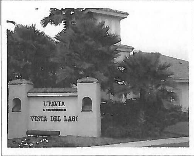
L'Pavia condominiums consist of 80 units. Shown here is the clubhouse for residents to enjoy.
