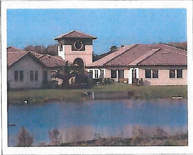
Lake View Office Park, located in the Jacaranda Commercial Center.
