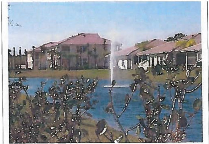
Vista del Lago consists of 50 home sites with like views as shown here.
