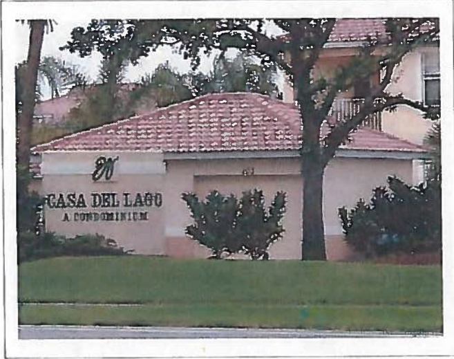
The Waterford Companies worked with city officials to keep designs consistent with the "Venetian Theme" on all of Venice Gateway projects.
